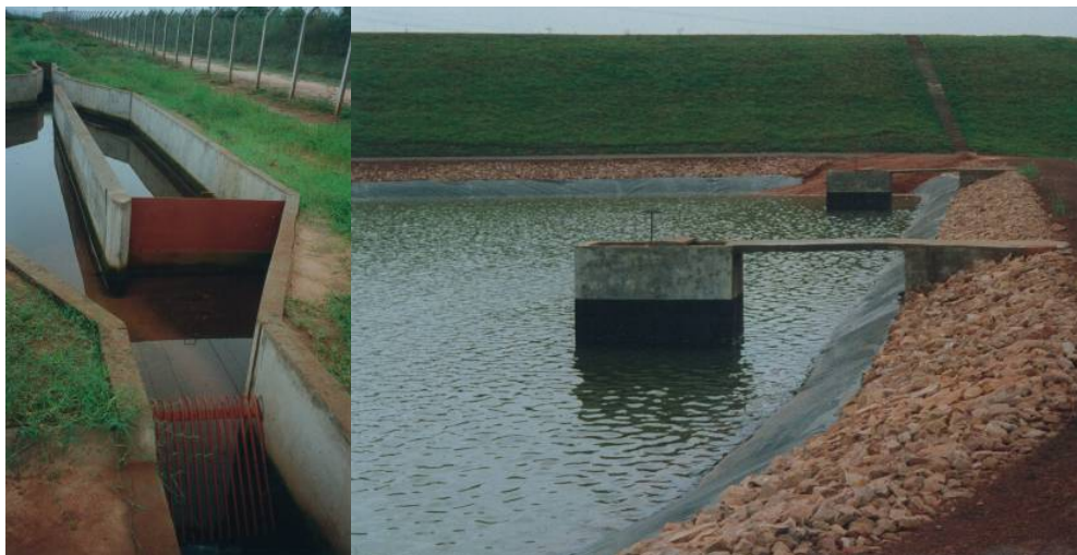
sewage treatment (top): grit chamber (1), pond discharge (2)
